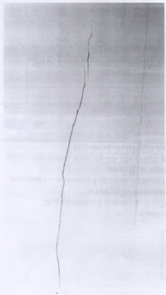
Vertical Cracks in Wall
