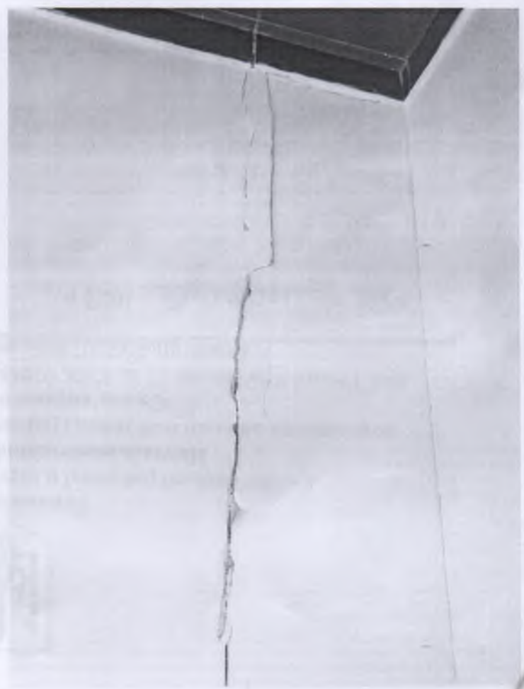
Vertical Cracks in Wall
